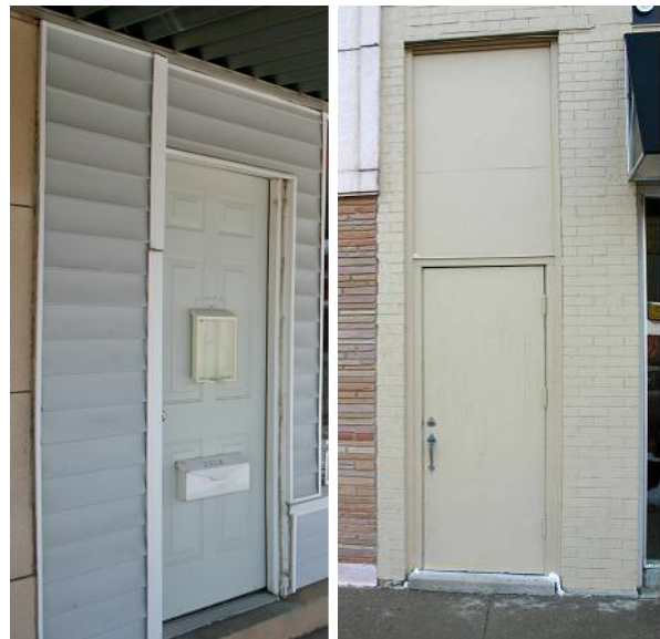
Inappropriate replacement doors and windows detract from the character of historic architecture and diminish the street-level appeal that distinguishes downtown Newton.
