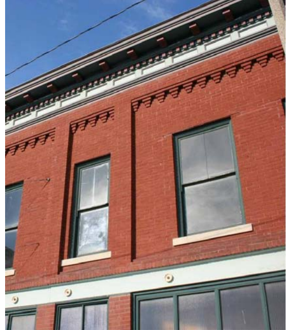
Features such as roof cornices with modillions and dentil moulding, as well as facade elements such as brick corbelling, should be retained. These should not be covered or removed.
