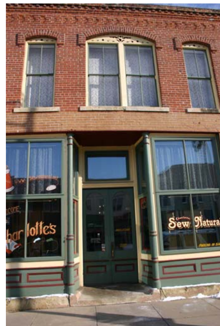
Cast-iron posts and wooden materials such as the ones that enframe these display windows are a common feature of historic storefronts. Existing storefront elements in downtown Newton should be retained.
