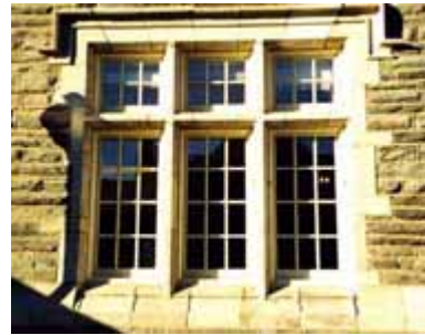
AFTER: Cleaned stonework and matching replacement windows after rehabilitation.
