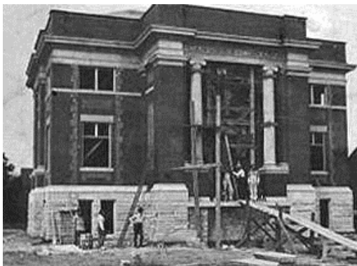
The Carnegie Library under construction, 1903.
