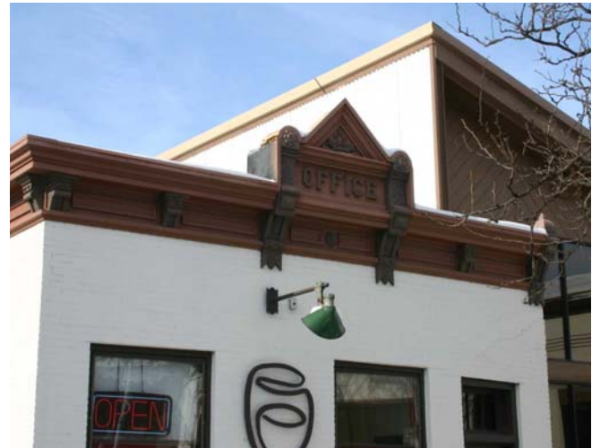
Appropriate light fixtures are unobtrusive and focused only on the area to be lit.
